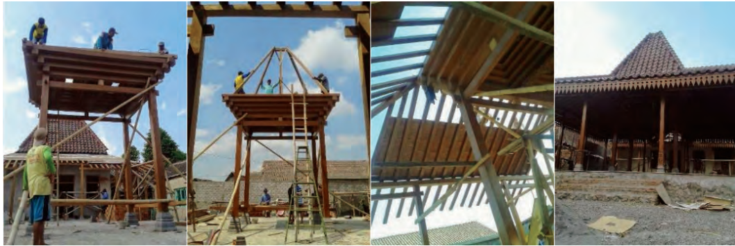
Figure 5 Process of Constructing Joglo (Source: Alvin 2019)
