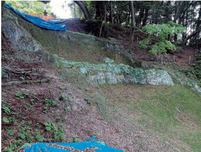
Figure 10 Reconstruction status as of June 2022 (Photo: Kanda town board of education)
